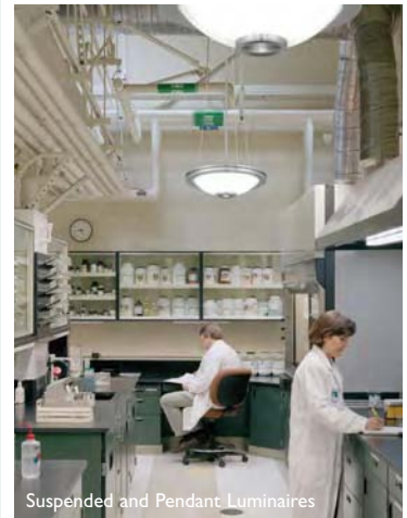
Suspended and Pendant Luminaires
